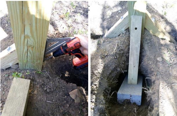
Arrange dirt to support the 16x8x4 concrete block at a 45deg angle centered and in tight contact with the bottom end of the 24in section. Reevaluate the vertical angle of the post and ensure that there is a slight angle rearward, even when applying pressure to the post forward. If necessary, apply rearward pressure to the post (releasing pressure against the block) while packing additional dirt under the block.
